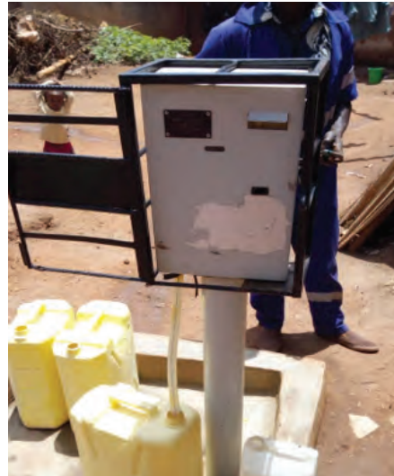
UPPB's Prepaid Water Standpipe
